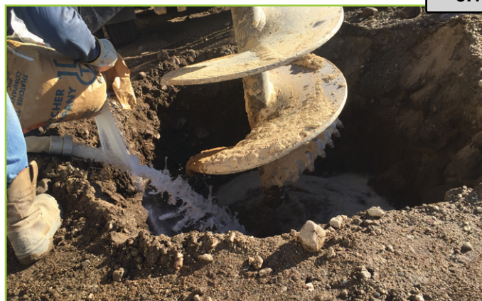
Auger drilling for the conductor casing placement
