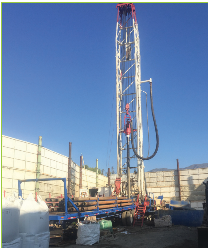
Borehole reaming for the Miragrand Well
