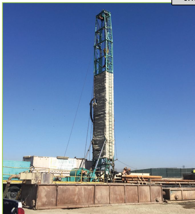
Pilot borehole drilling for CDA-II-12
