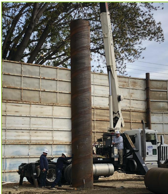
Installation of conductor.
