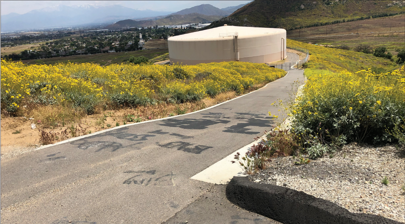
Access road looking east at Reservoir 2-3
