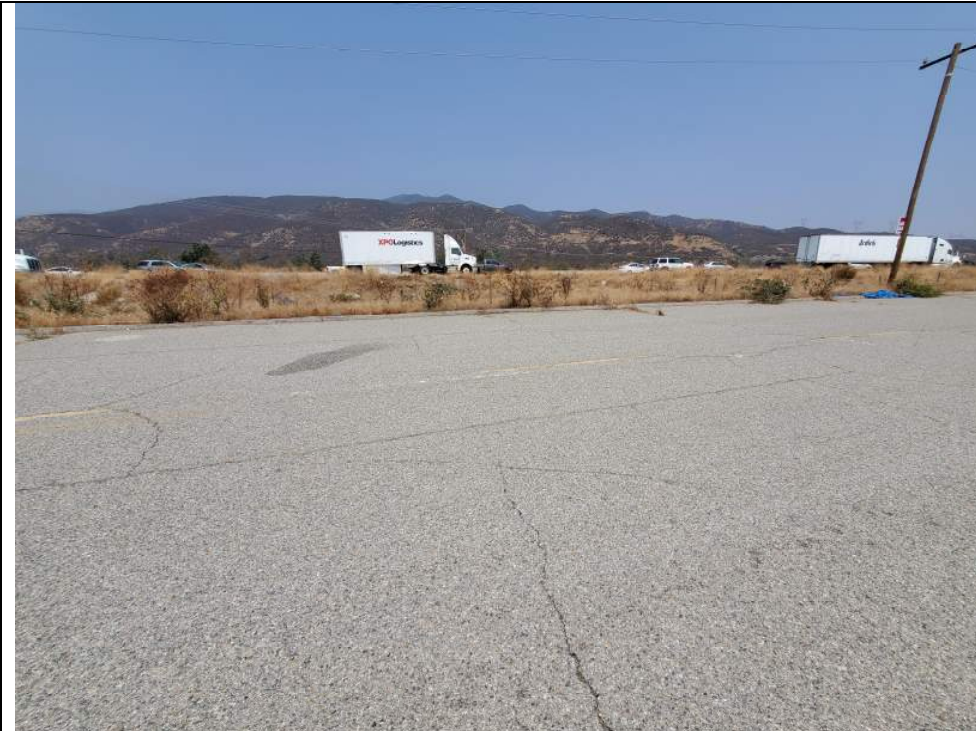
Photo 5. South side of Project alignment; looking northwest toward I-15 from Citrus Avenue.
