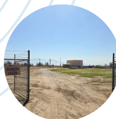
Lord Ranch Facilities Projects: Reservoir, Pump Station and Site Improvements
