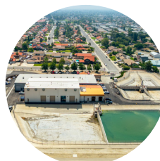
Oliver P. Roemer Water Filtration Facility Expansion
